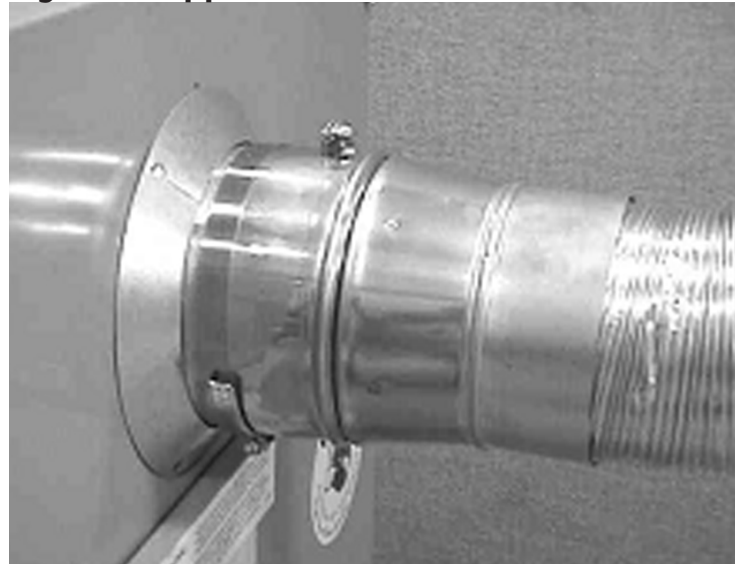
Figure 6 - Appliance Connector w/ Test Port
