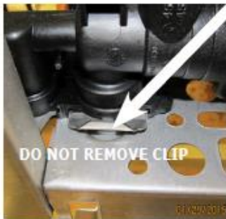
LEFT SIDE CLIP - INSIDE BOILER JACKET
