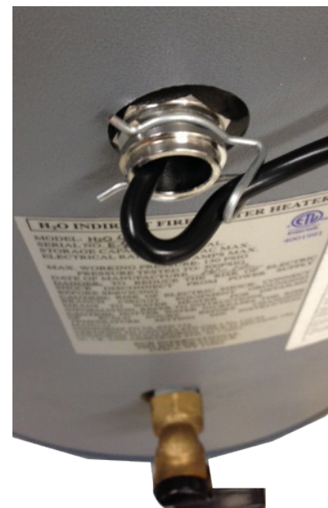
Figure 3 - Sensor Wire Secured to Well With Clip
