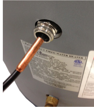
Figure 2 - Secure Sensor Wire to Well With Clip
