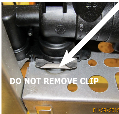
LEFT SIDE CLIP - INSIDE BOILER JACKET
