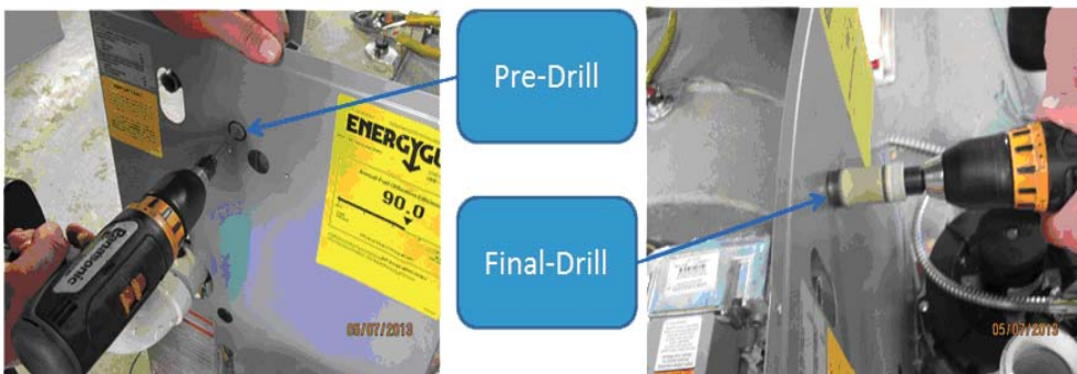
Figure 12 - Drill Hole For Junction Box
