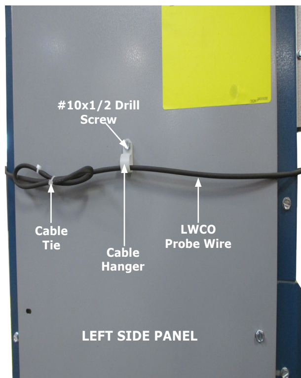
Figure 2 - Low Water Cutoff (LWCO) Probe Wiring
