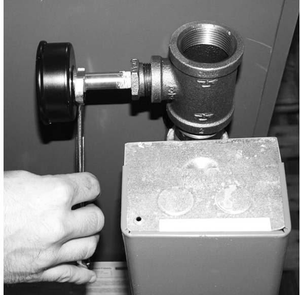
Figure 9 - Tighten Gauge With Crescent Wrench
