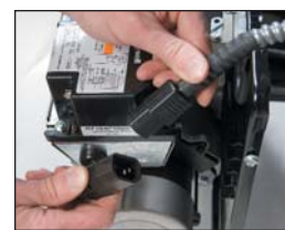
Beckett burner with plug 'n play connector
